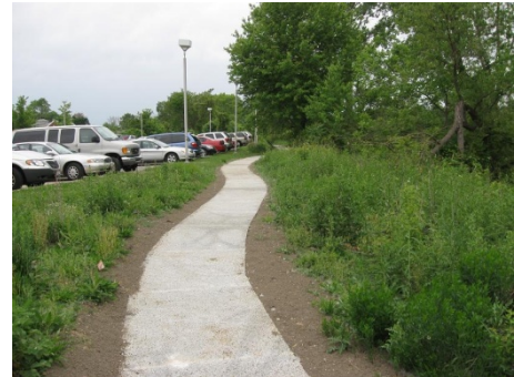
Pervious concrete path at Lutheran Homes
